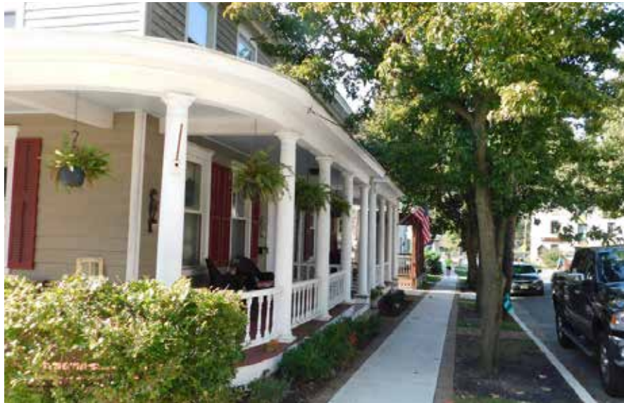
Well preserved porches with Main Street frontage
